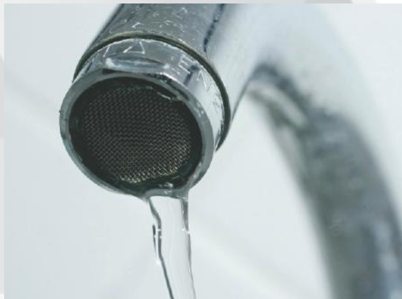
Water Tap Off Point
